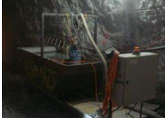
pump held in reserve. The pump is frequency-controlled and regulated using a submersible pressure probe. If the water level rises, the speed is increased; when the water level falls, the speed is reduced. This type of control was chosen so that a very small pump container can be used which can be easily replaced after each new tunnel section. A model KTZ47.5 pump is built into the drainage water treatment.
