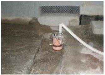
The incoming muddy water is pumped out with a total of ten model LCS1.4S pumps. These are abrasion-resistant residual water pumps, which pump out the water down to a height of 1mm. The builtin check valve allows continuous suction operation; no personnel is needed to monitor the pump operation.
