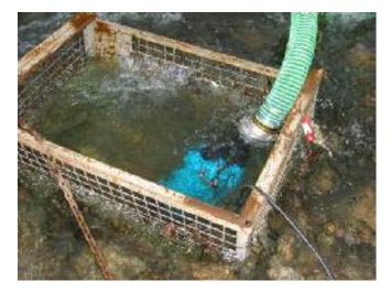
A pump in the KTZ series was used, secured with a steel cage. Particular value was placed on operational safety, which was guaranteed at all times thanks to the quality of our pumps.
